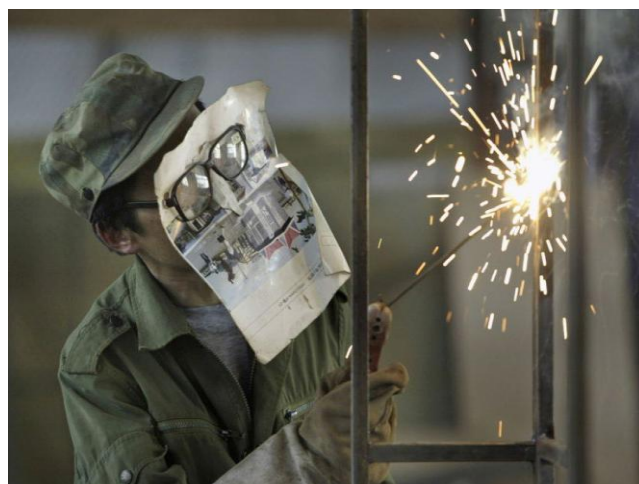
A worker performing hot work in a highly unsafe manner
